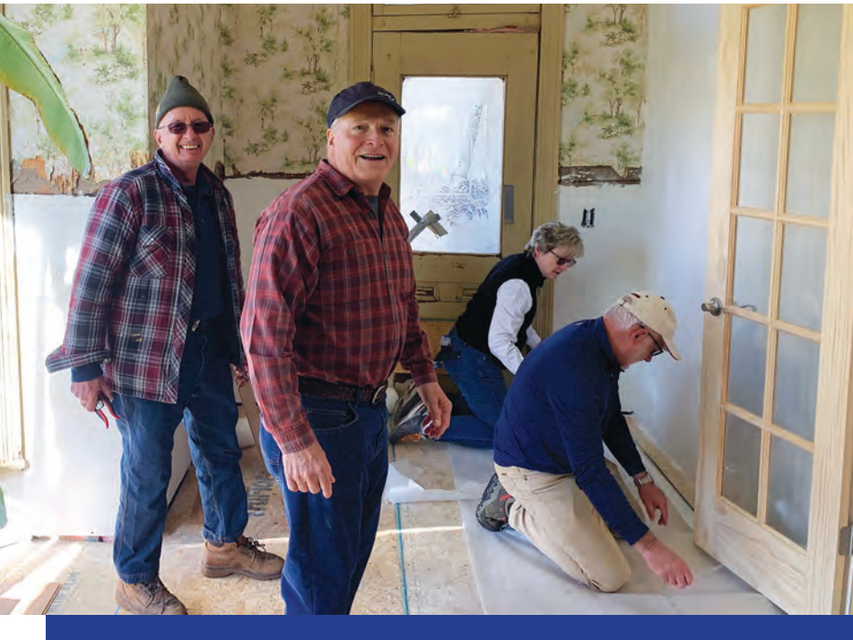
Working at a damaged home in Waverly, TN in March
